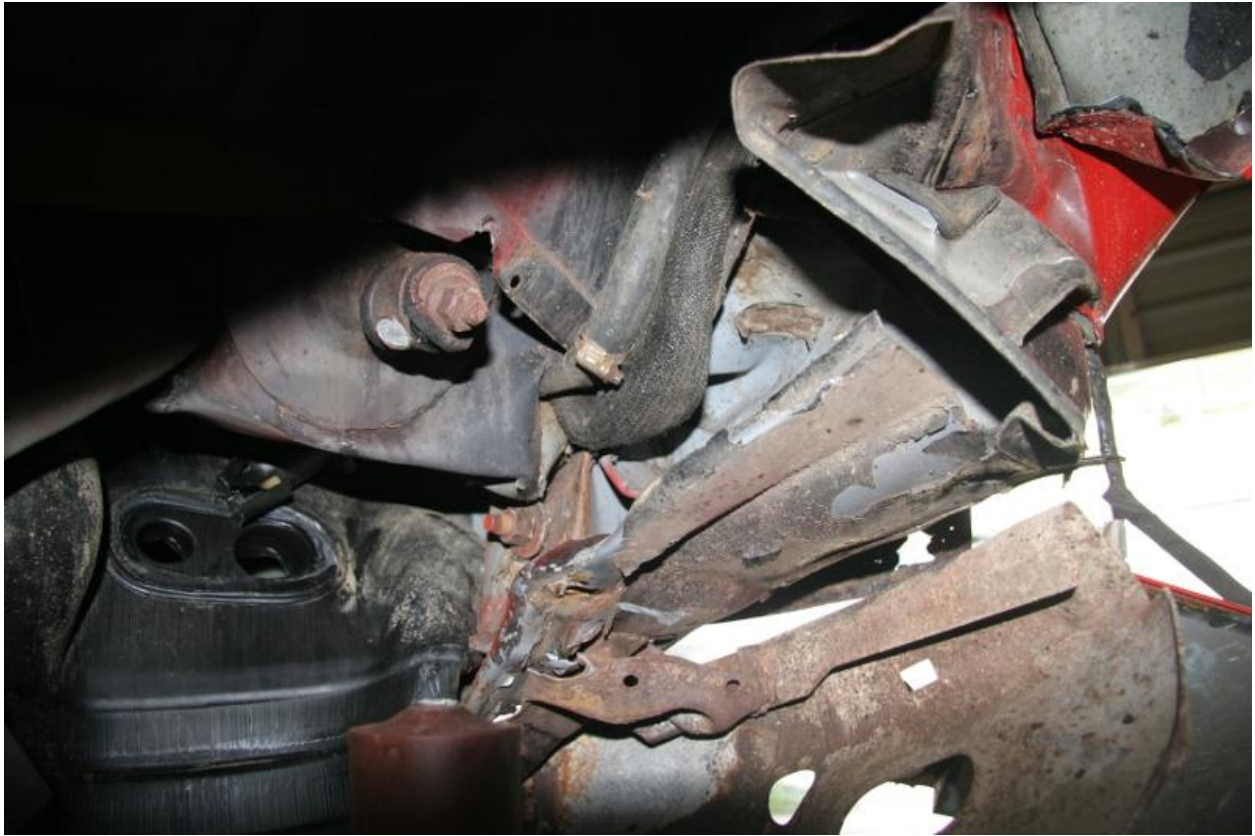
Exhibit C – Fuel Tank Connection Where Filler Tube Pulled Loose
