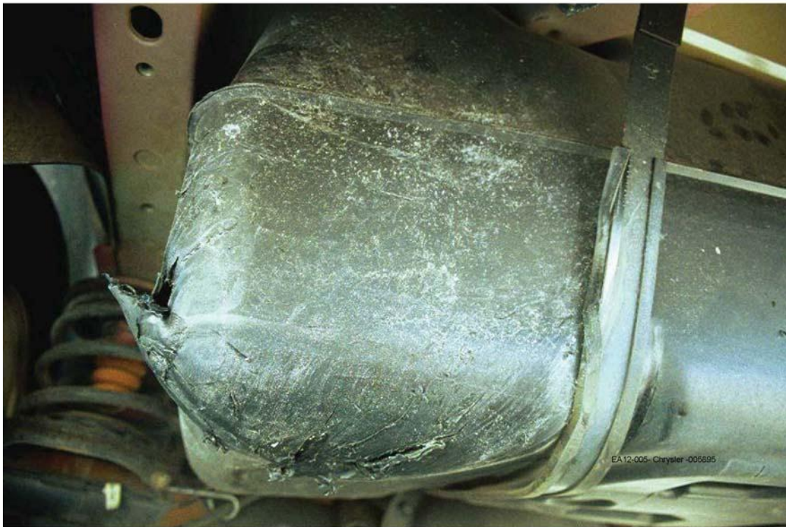
Figure 4 Rear Impact Damaged 2002 Liberty Fuel Tank.
