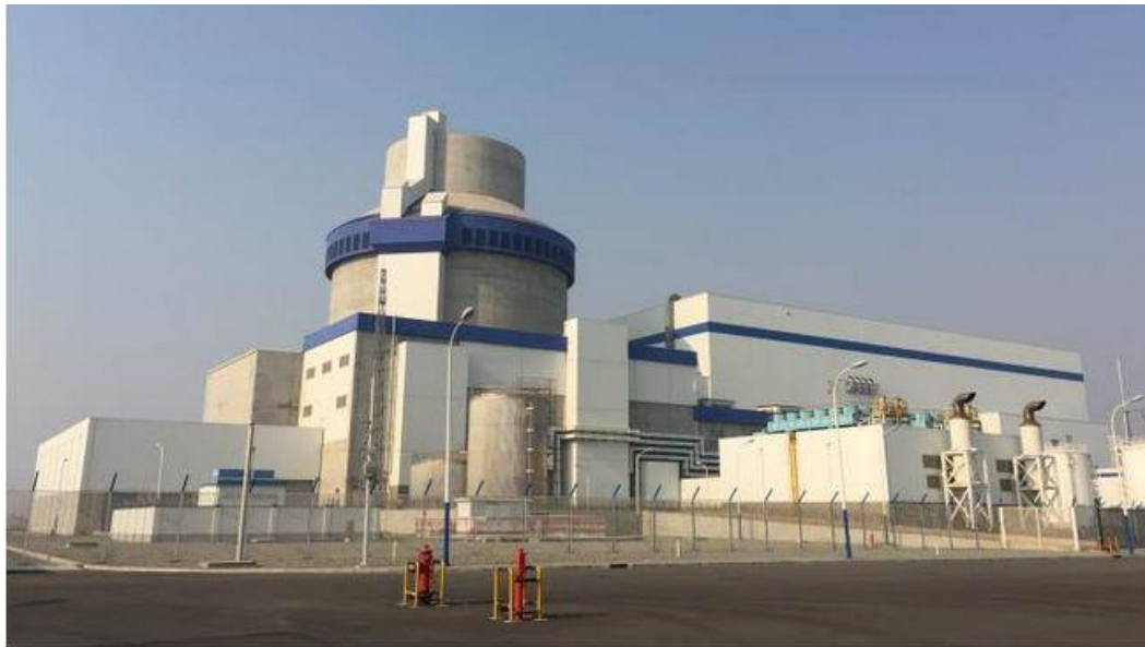
Unit 1 of the Haiyang plant (Image: Westinghouse)
