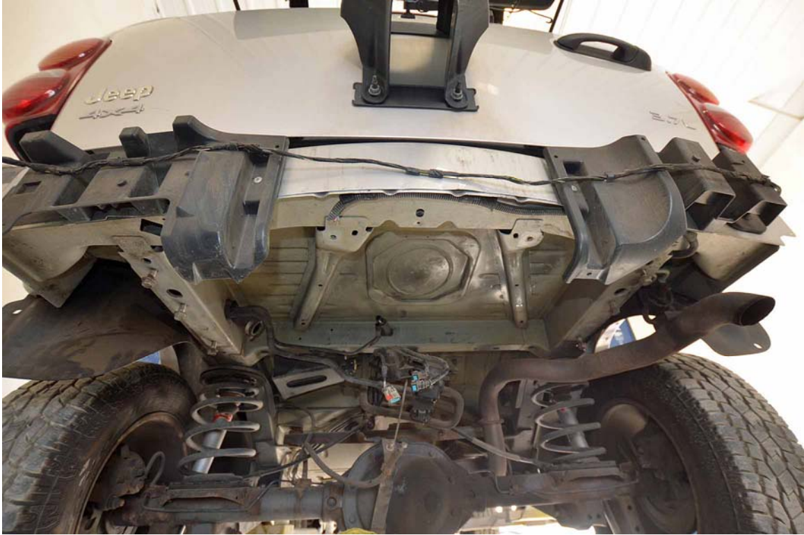
FIGURE 25. 2003 Jeep Liberty Fuel Tank Removed
