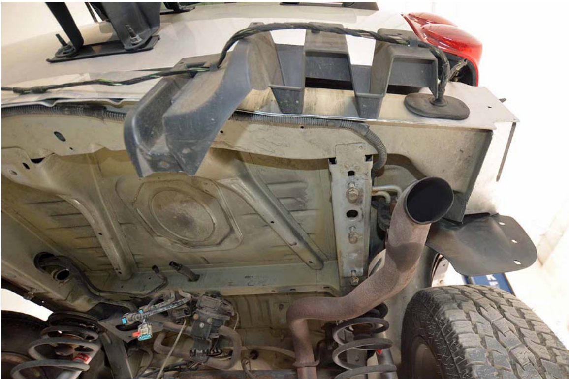
FIGURE 26. 2003 Jeep Liberty Fuel Tank Removed
